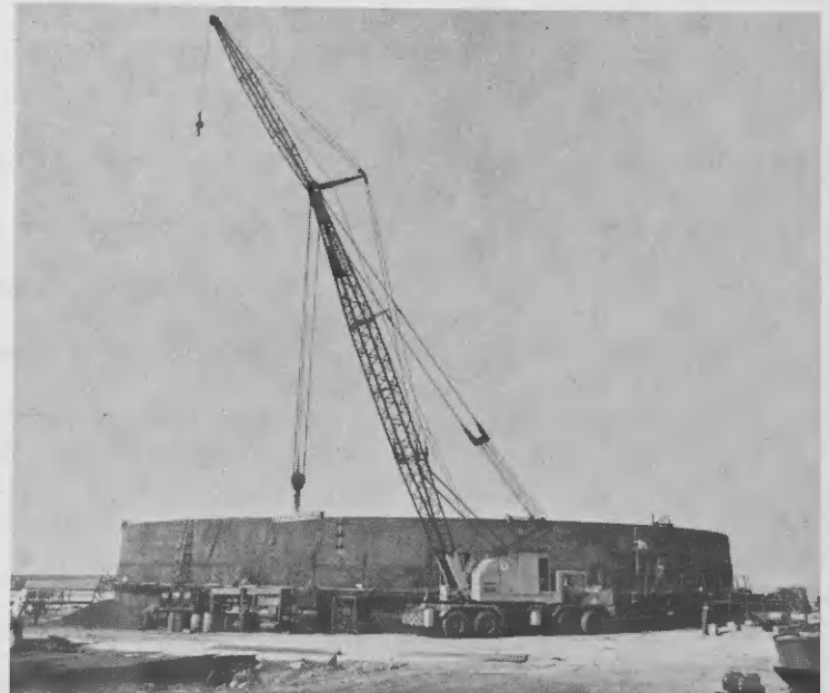
New deballasting Tank 402 will be six times the capacity of the present tank of 30,000 barrels.
